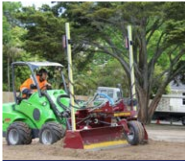
Laser levelling underway
